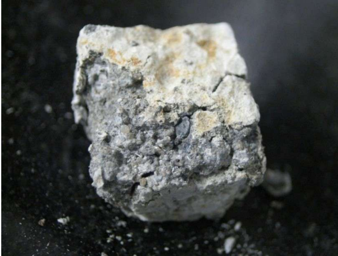
Figure 5.35: Deteriorated strength-tested sample after 84 days of exposure
